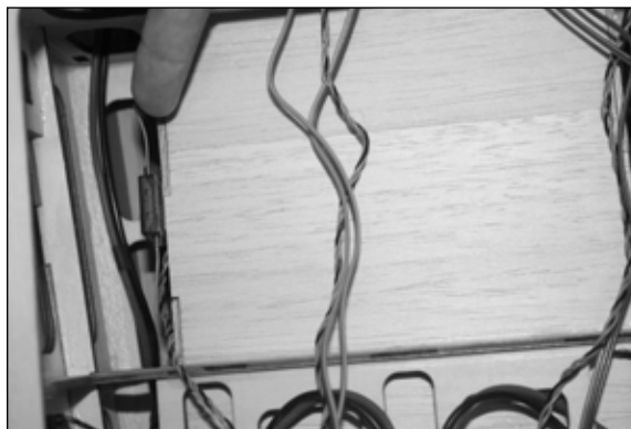
Location of Satellite receiver3 - front of the tank and on the left vertical side.
